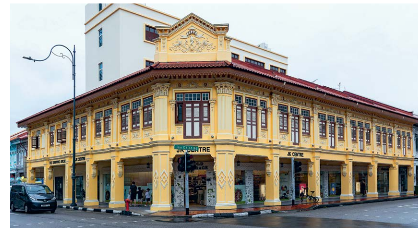
The distinctive yellow shophouse along Joo Chiat Road, whose design features a blend of Chinese and Western elements.
