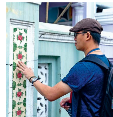
A tour participant admiring the intricate tiles on the facade of a house at Koon Seng Road.
